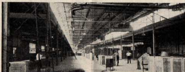
From this long assembly room Crosley sets can be loaded on waiting freight cars at the rate of 580 per hour.
